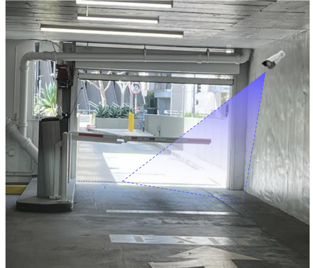
Exit camera is placed above the exit drive lane to record vehicles as they exit from the facility
