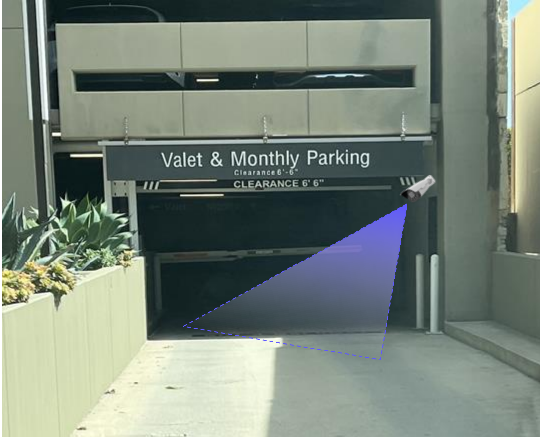
Entry camera is placed above the entry drive lane to record vehicles as they drive into the facility
