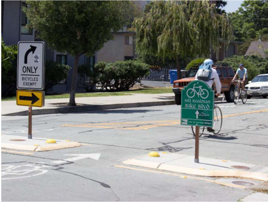
FIGURE 45: TRAFFIC CALMING DIVERTER – BIKE BOULEVARDS
