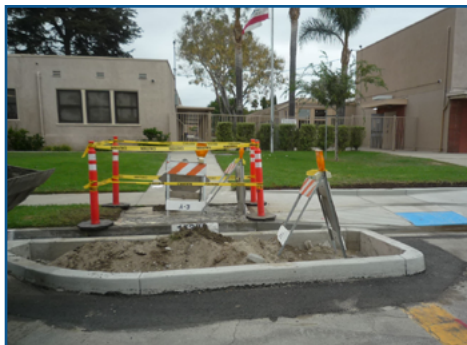
Island to install RRFB and reduce speed.
