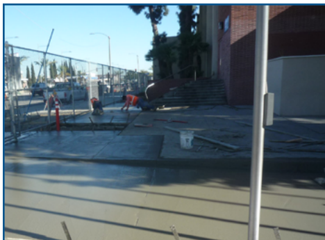
Pouring concrete for sidewalks and ADA ramps.
