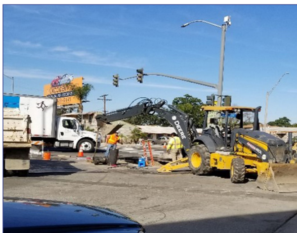
Cast Iron Main Replacement
