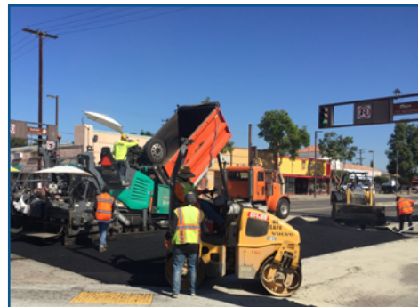
Resurfacing street with asphalt.
