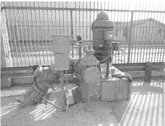
WELL SITE: EXISTING 125 HP WELL PUMP.
