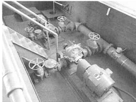
BOOSTER PUMP STATION: 25 HP (LEFT) & 75 HP (RIGHT)
