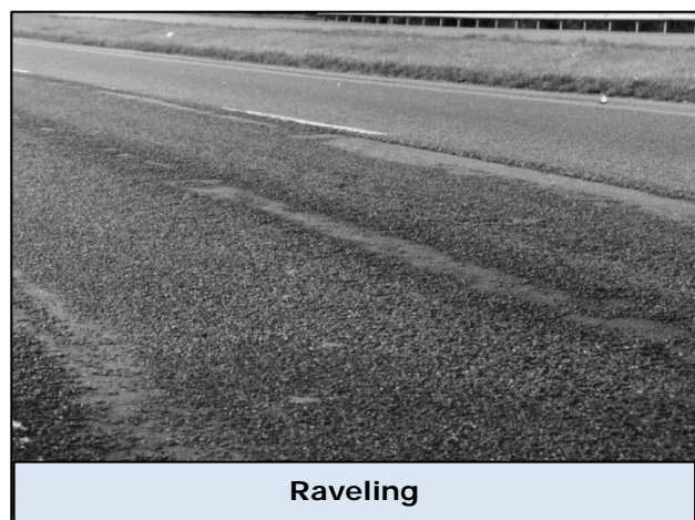
Figure 1: Common Distresses for AC Pavement
