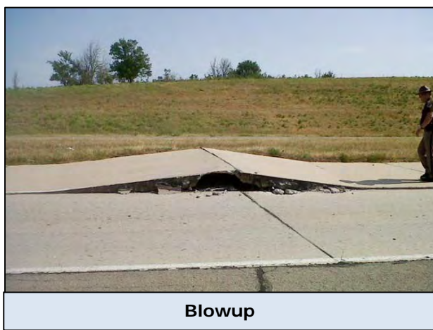
Figure 2: Common Distresses for PCC Pavement
