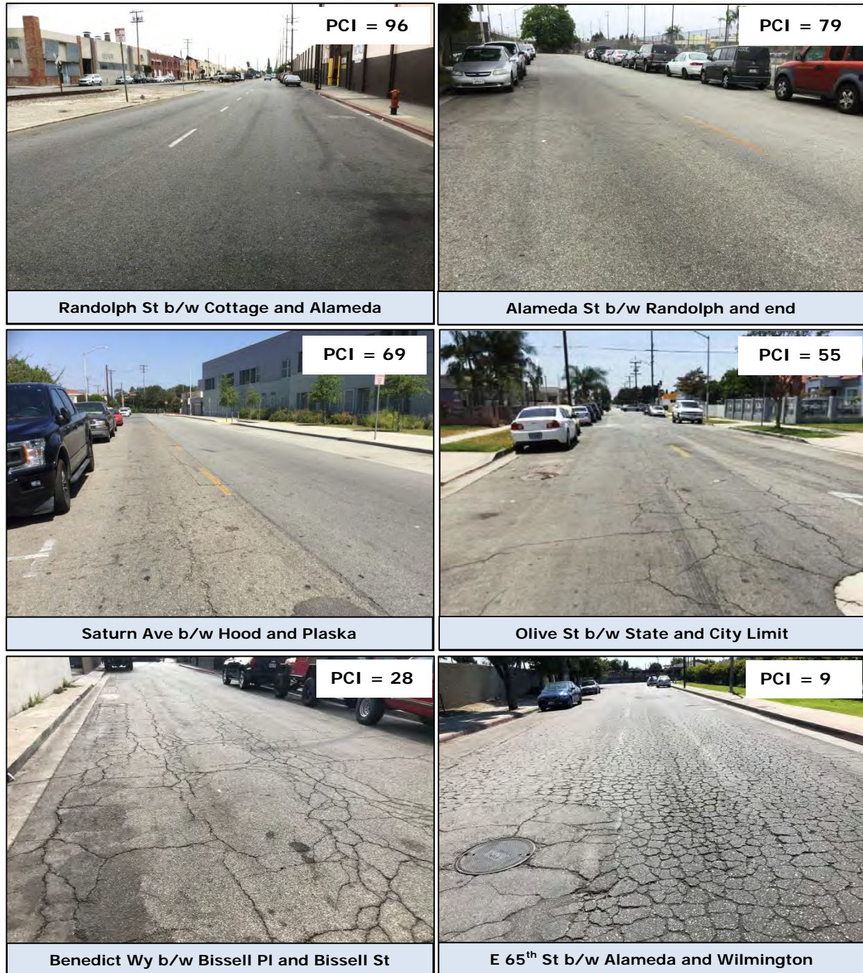
Figure 4: Examples of AC Streets with Different PCIs
