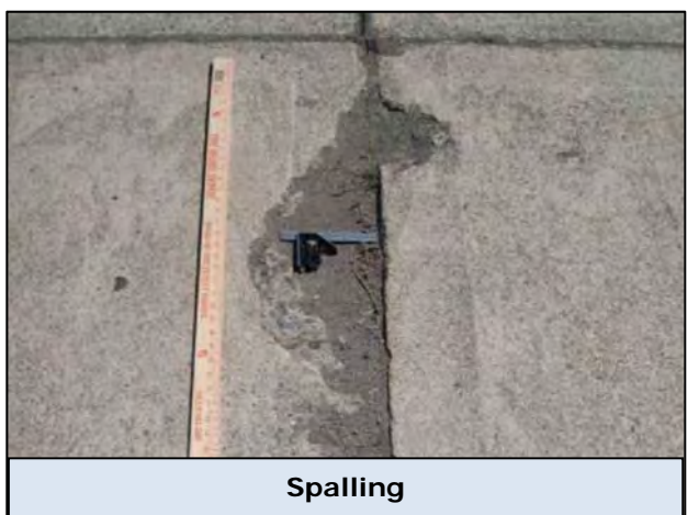
Figure 2: Common Distresses for PCC Pavement
