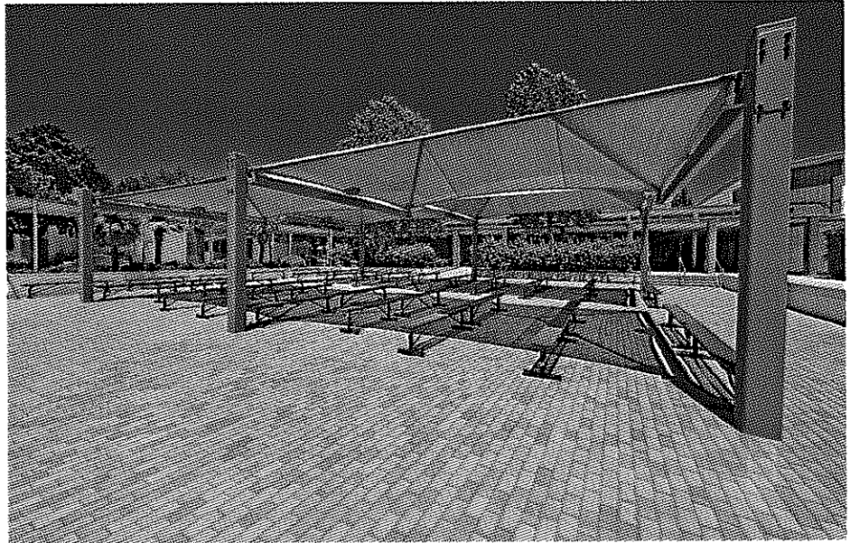
Shown: Tuscan Holland installed in a running bond pattern.
